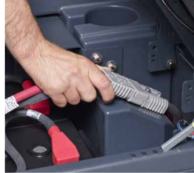
3. Check battery cables are well connected together.
